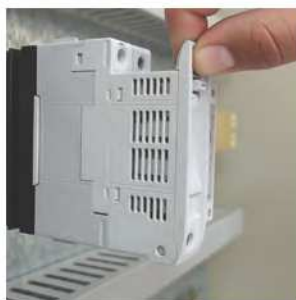
1. Preparation for opening fuse holder
