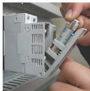
3. Removal or Insertion of fuse
